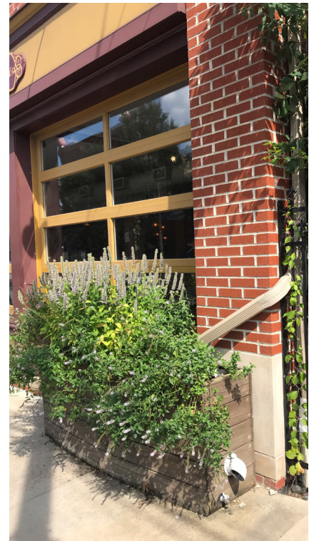
This rain planter collects water from the building's downspout and helps grow flowers. The planters are sustainable because in a heavy rainfall, water is retained in the planter instead of running immediately into the storm sewers and causing flooding or stormwater overflows.
