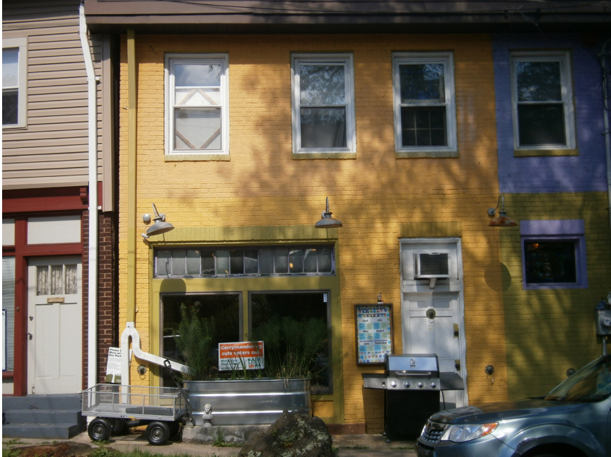
This building on South Trenton Street most likely was altered by adding a storefront. Previously, the property likely was a rowhouse.
