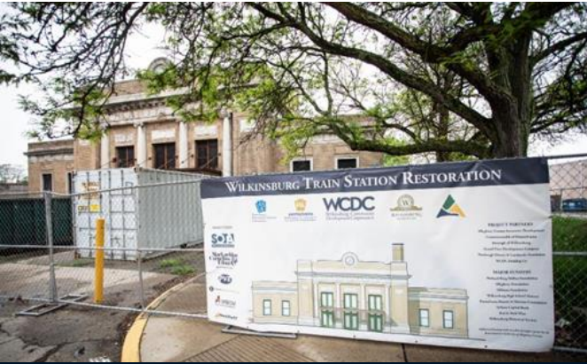
Renovated community anchors
