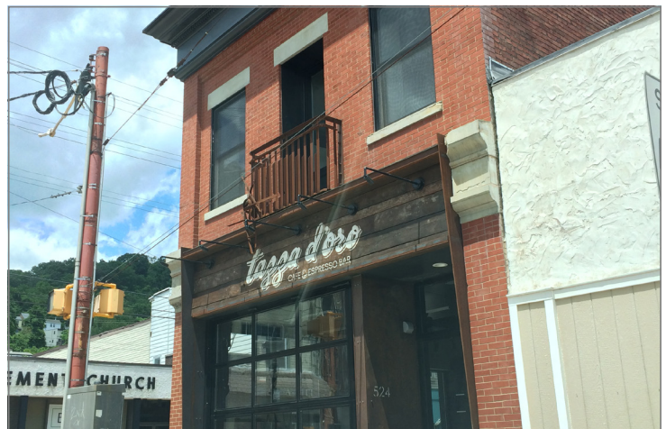
↑ TAZZA D'ORO IN MILLVALE, PA IS AN EXAMPLE OF STRATEGIC RENOVATION OF AN EXISTING BUILDING AT A KEY INTERSECTION.
