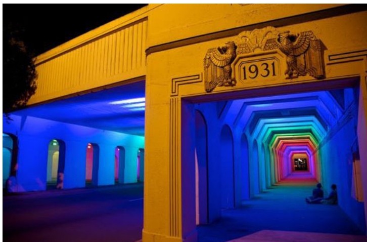
EXAMPLE OF AN IMPROVED HISTORIC UNDERPASS
