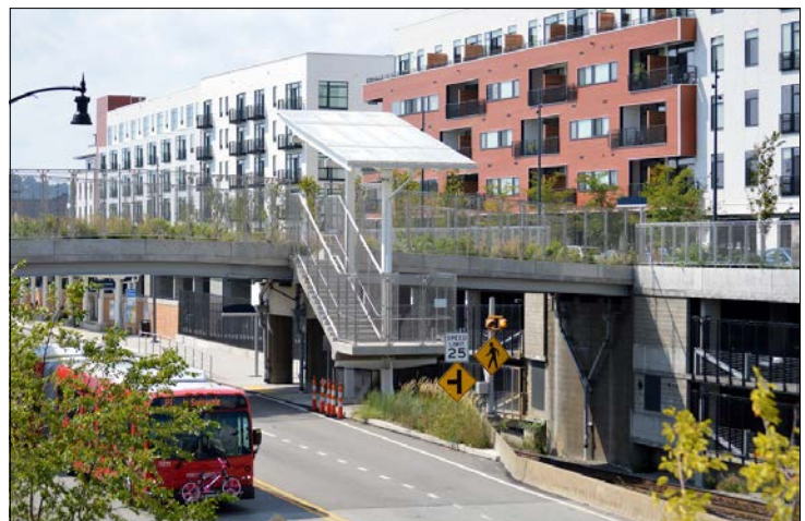
↑ EAST LIBERTY BUSWAY PEDESTRIAN BRIDGE
